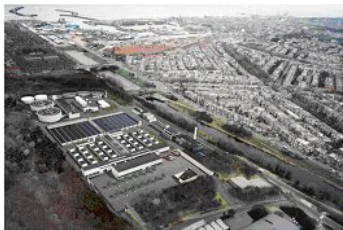
Houtrust waste water treatment plant
