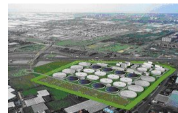
Harnaschpolder waste water treatment plant
